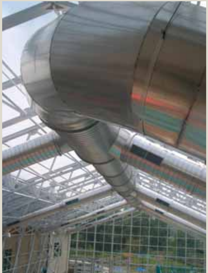
The new Hockessin Athletic Club in Hockessin, Del., has more 522 linear feet of aluminum spiral ductwork made by Wm. H. Brady Inc. of Elkton, Md.
